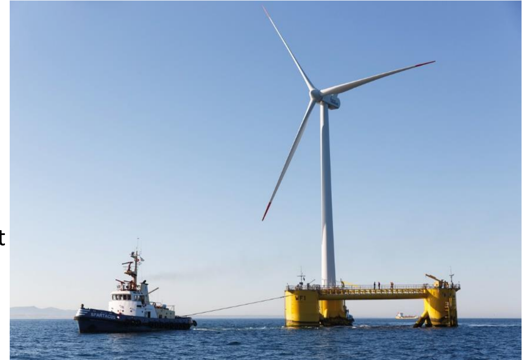
PPI WindFloat prototype towed in Portugal
